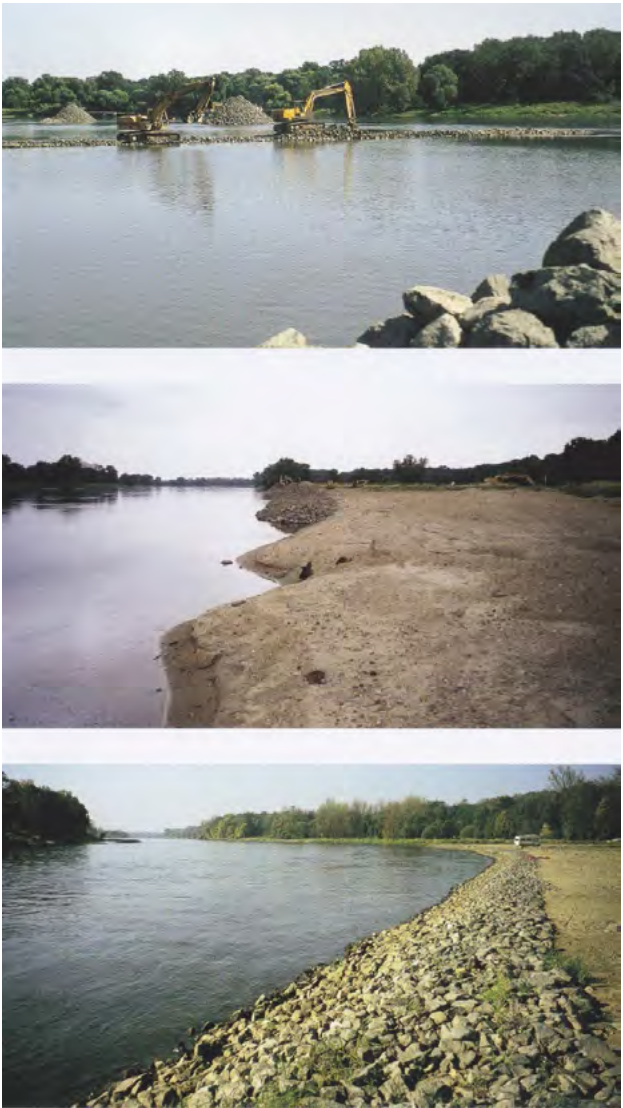
Fig. 16: Until the dredgers came and drove new groynes into the river (above), shading of the banks also began in many places (center) and was completed at this section (bottom) (Dörfer 2000).
